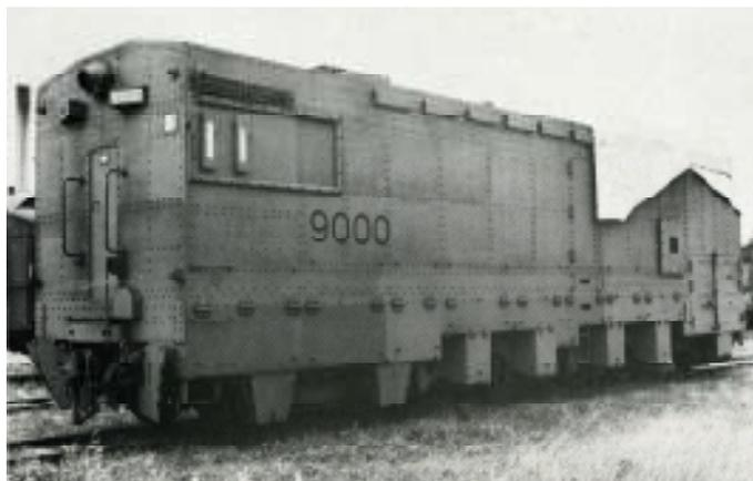
The 9000 sheathed in armour plate for wartime service, one unit of the locomotive was ungainly; it never saw active duty.
